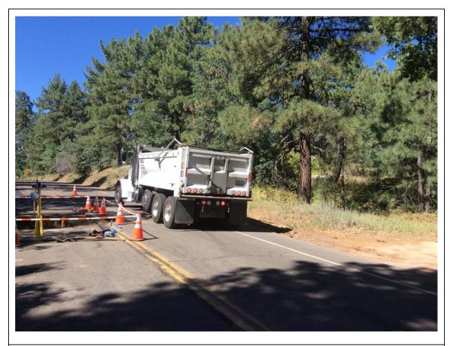
**Photo 1:** Haul truckloads of spoils from trenching activities on C 440 were observed to be covered while traveling on public roadways in accordance with APM AIR-02.
