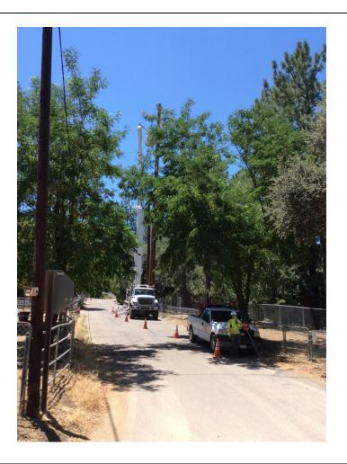
**Photo 6:** A crew was observed conducting overhead work at Pole Z173157 (TL 629A). Cones, signage, and flagpersons were used to direct one-way traffic around the work area in accordance with the TCP (APM TRANS-05) and APM TRANS-02.
