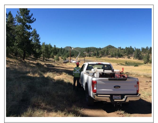
**Photo 4:** A Dedicated Fire Patrol was present and equipped with at least 150 gallons of water with pump and hose during conductor dead-end activities at Pole P45308 (C 440) in accordance with the CFPPP Fire Prevention Matrix for conductor replacement of de-energized lines off USFS land with an Elevated FPI (MM FF-1).
