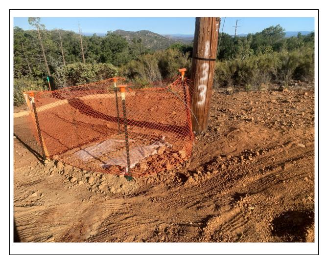
**Photo 2:** A direct-bury pole hole at Pole P258558 (TL 626 Conversion South (C 79B)) was observed to be covered to prevent wildlife entrapment in accordance with MM BIO-23.
