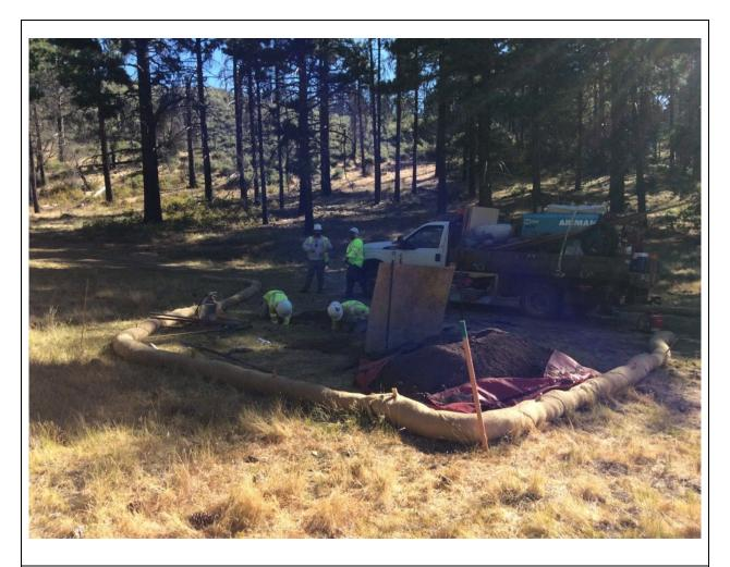
**Photo 5:** A crew was observed installing grounding rods and wire at Pole P259909 (C 440). Erosion control BMPs at the site were observed in good condition in accordance with the ECP, the SWPPP, and APM HYD-09.
